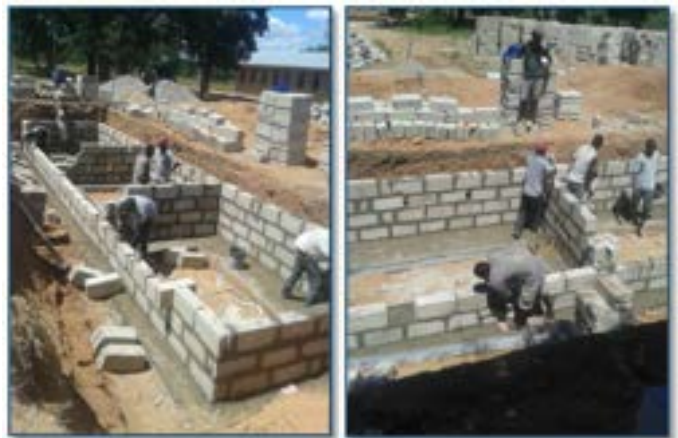
Current work on the new toilet
